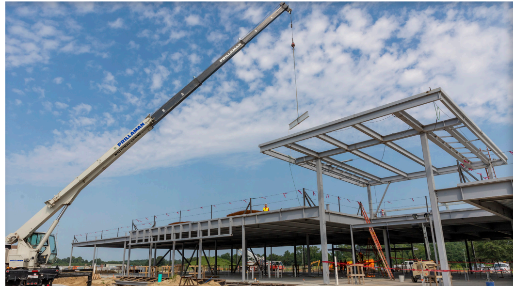
The signed beam is put into place at Riverside Smithfield Hospital.
